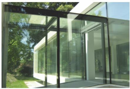
The forming of aesthetic and comfortable living space has resulted in using large, several square meters in surface, glass constructions. Because of these changes in the wall/glass ratio and the building constructions following the high lagging standards of buildings, the loss of heat, even with glass structures produced using state of art coating, is the highest at the windows and the doors.
